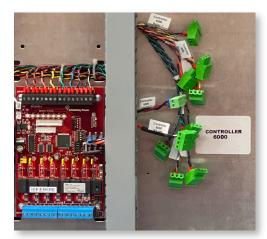
Consistent color-coded twisted pair wiring
